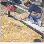
ON THE ROOF, Charron removes the shingles from the area where the skylights are to be installed using the nail as a guide. The shingles are set aside since some will be reused to finish
