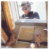
IN THE ENSUITE Blondin uses scraps of drywall held in position to ensure a proper fit, leaving the appropriate gaps for tolerances
