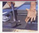
INSTALL THE step flashing using the %" nails provided
