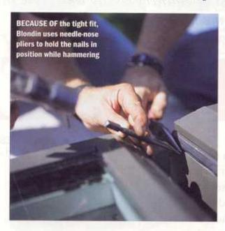
REPLACE FRAME cladding parts, starting at the bottom of the skylight frame
