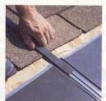
INTERLOCK HEAD flashing sections with the slide strip and then hammer to lock
