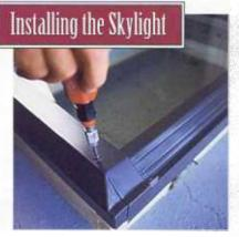
REMOVE THE skylight kit from the box and, following the instructions, disassemble the cladding parts from the frame
