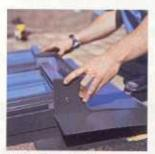
TEST-FIT them first, then position the head flashing sections against the skylight frame
