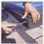
MAKE SURE top frame cladding is placed in position. Fasten with original screws
