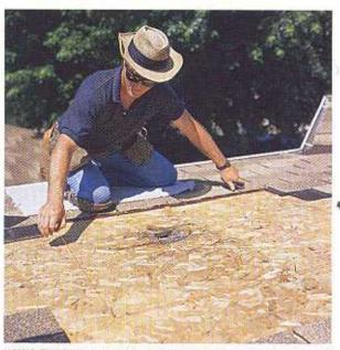
USING THE NAIL as a guide, level, square and mark the opening for the skylight with a chalk line snapped on the roof deck
