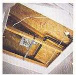
REDIRECT ANY electrical wiring and plumbing before cutting the hole in the roof for the skylight
