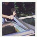
POSITION MIDDLE gutter and attach to side frame with nails
