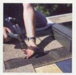
REPLACE THE shingles and nail them into the roof decking
