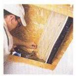
**BUILD BRACES between the** rafters for extra support. Hammer a nail up through the roof to mark the roof opening
