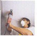
MAKING THE cut from the inside (using a reciprocating saw) makes catching the drywall cutout easier
