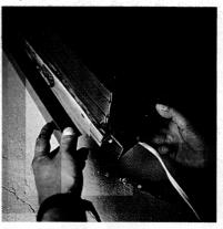
**REMOVE SIDES, then top and bottom** before installation. Paint or stain the skylights now, prior to final installation
