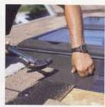
**FLASHING PARTS must** overlap a minimum of 31/4"
