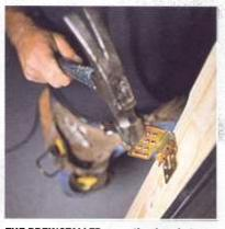
THE PREINSTALLED mounting brackets are tapped and locked into position for installation. Location depends on roof material
